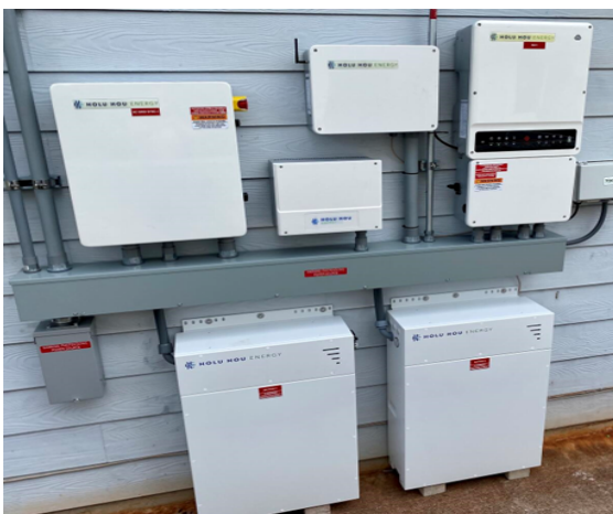
A HoluPower xP system consisting of 9.6kW of AC power with 16.4kWh of energy storage.
